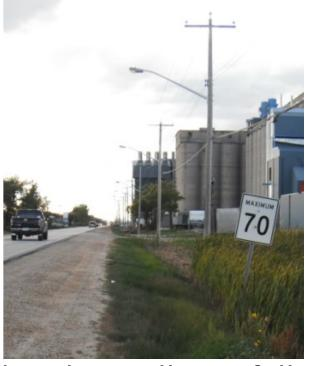
Signs at extreme heights will not fall within a driver's line of sight. The above are speed limit reduction signs and are not compliant with standards.
