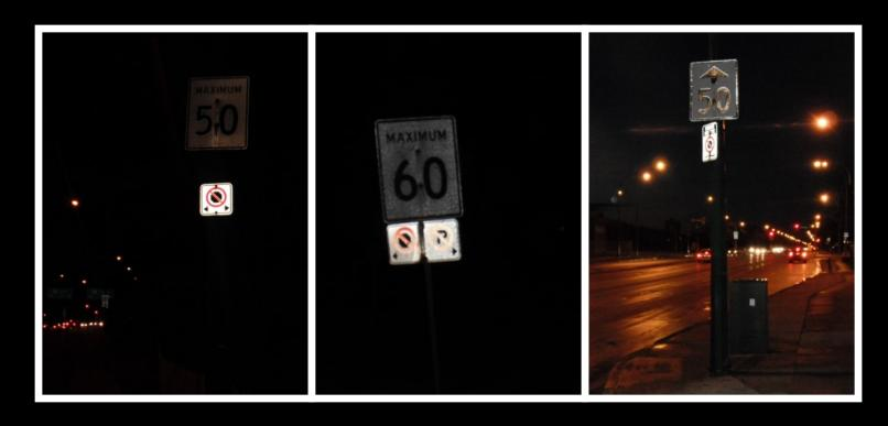
Some speed limit signs in Winnipeg have little to no reflectivity while other signs, often on the same pole, are fully reflective. The first two of the above examples were before photo radar locations that are used for night time enforcement.
